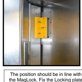
The position should be in line with the MagLock. Fix the Locking plate to the leading edge. 10mm packer provided if needed. Use Lock Thread on all fixings.
