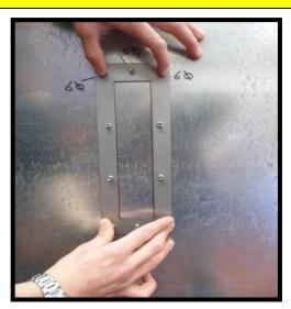
Disassemble template from Maglock assembly first. Hold the support template onto the car wall and mark out the drill holes and hole cut out
