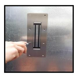
Now install the MagLock as shown. **Use Lock Thread on all fixings.**
